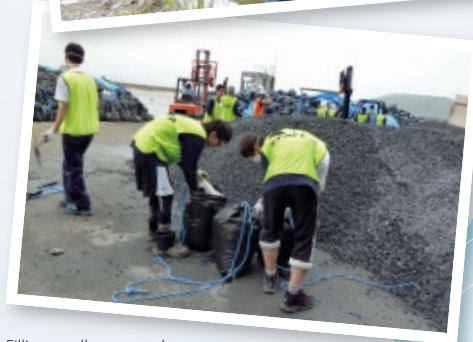
Filling sandbags near the port
