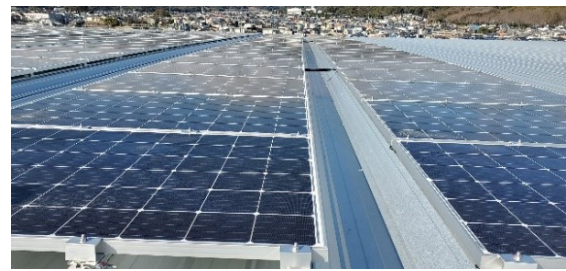
Solar power panels installed on the roof
