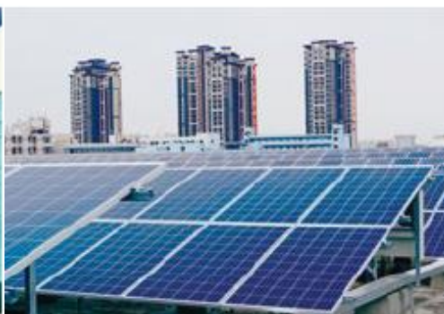
Solar power panels installed on the roof
