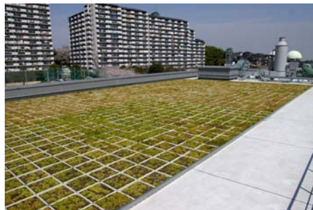
Osakasayama Site (rooftop greening)
