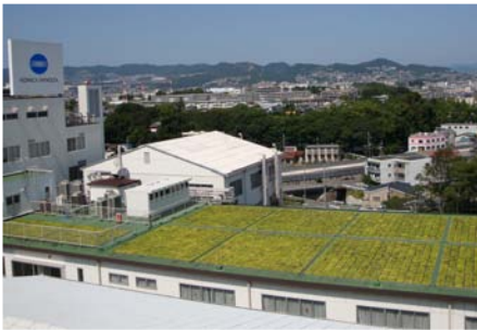
Itami Site (rooftop greening)
