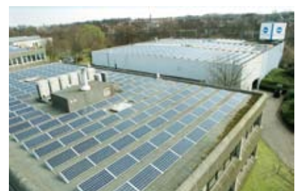
Solar panels installed on the roof of the company building
